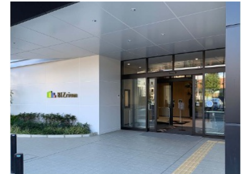
"BIZrium NAGOYA" Sub Entrance
